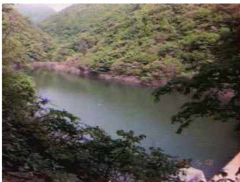
Fig.10 Large inundation area (Maenokawa River dam)
