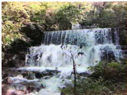
Fig.14 Sarabuchi dam in old style
