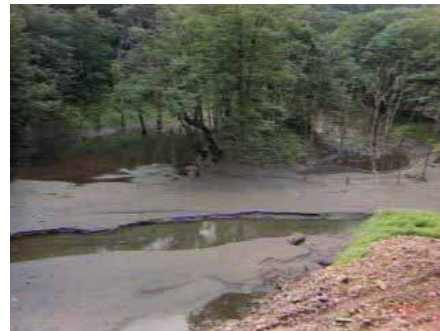
Fig.9 Water pathway in the sediment (Kanosawa River 4th dam)
