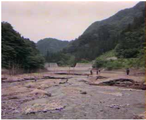
Fig.6 Water pathway among accumulated sediment (Wasada-gawa River 2nd dam)
